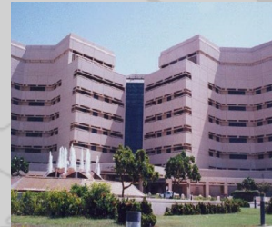
Khomees General Hospital IBS DAS and Civil installations.
