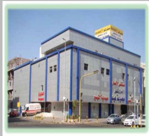
Ansar Hospital (IMD 174) IBS DAS and Civil installations.
