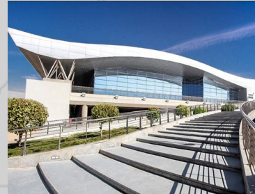
Riyadh International Convention & Exhibition Center IBS Das installation
