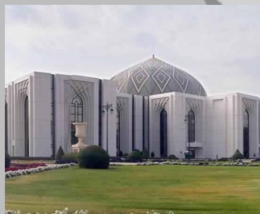
Alyamama palace IBS Das installation
