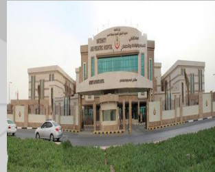
Maternity & Children Hospital Khomees IBS DAS and Civil installations.
